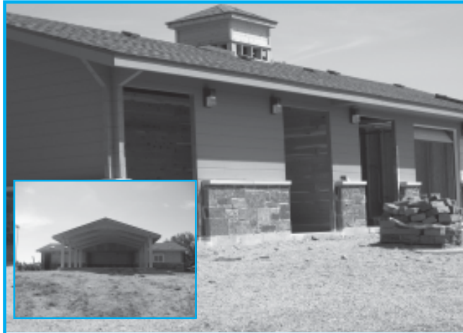
Under construction: a new pavilion at Village Green Park.
